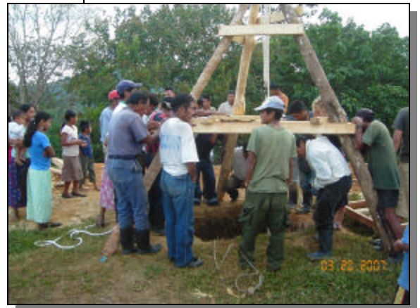
The well and caisson-lowering tripod is inspected
