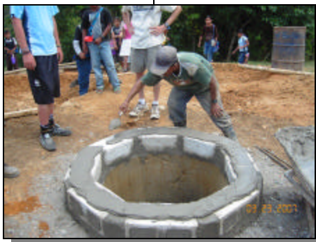
Clockwise from bottom left: the finishing touches before the well is covered and the pump installed; it took the strength of many men to lower the heavy caissons; engineering student Grant Ovist turns fire-fried pancakes; children were curious about the caissons and engineering student Juan Morinelly; entertainment included traditional dance by the schoolchildren.
